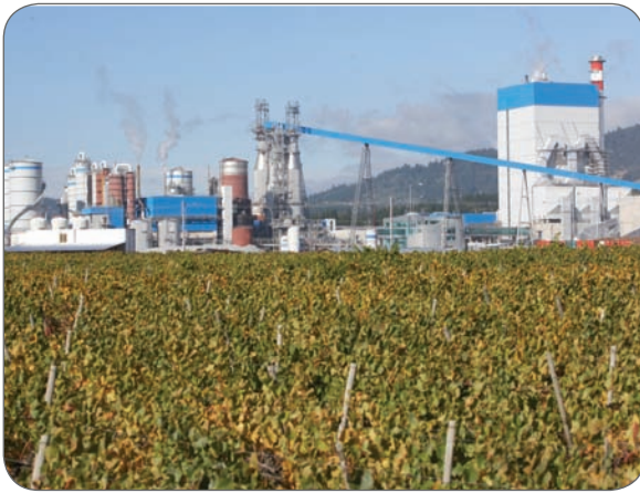
The Celulosa Arauco Mill at Nueva Aldea, Chile, met its safety, environmental and quality goals after start-up.
