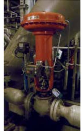
*As part of a turnaround, Emerson-certified service technicians installed new stainless steel FIELDVUE DVC6200 instruments to Fisher rotary and sliding stem control valves.*
