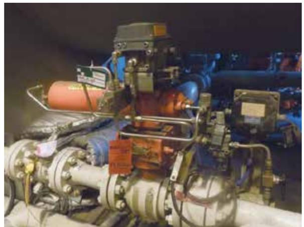
*For an offshore platform, Emerson-certified service technicians modified the instrument tubing and added Fisher FIELDVUE DVC6200 digital valve controllers to a competitor's shutdown and blowdown valves.*
