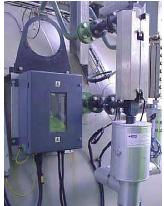
Figure 1: Hydrastep installation
