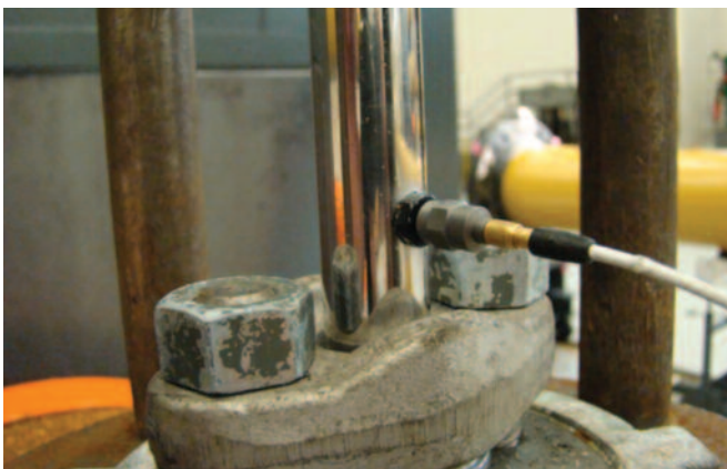
Typical mounting of accelerometer to valve stem.
