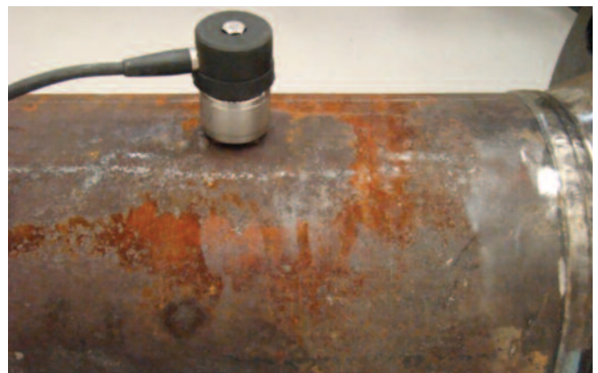
Magnetic mounting of an accelerometer to a pipe wall.
