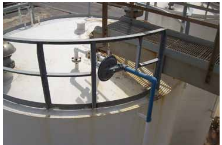
Fisher Type Y693 Tank Blanketing Regulator Installed at a Major U.S.A. Chemical Plant
