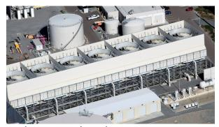
Wireless now provides cooling tower riser temperatures which are used in the efficiency calculation to confirm the fans are running at correct speeds. This enabled the power plant to stop over-compensating, which has improved thermal efficiency.
