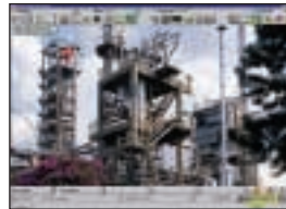
EMERSON'S CONTROL STUDIO
