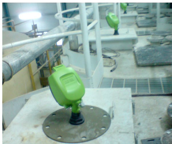
The 3D Solid Scanners were installed on all the solid material silos in the mill.
