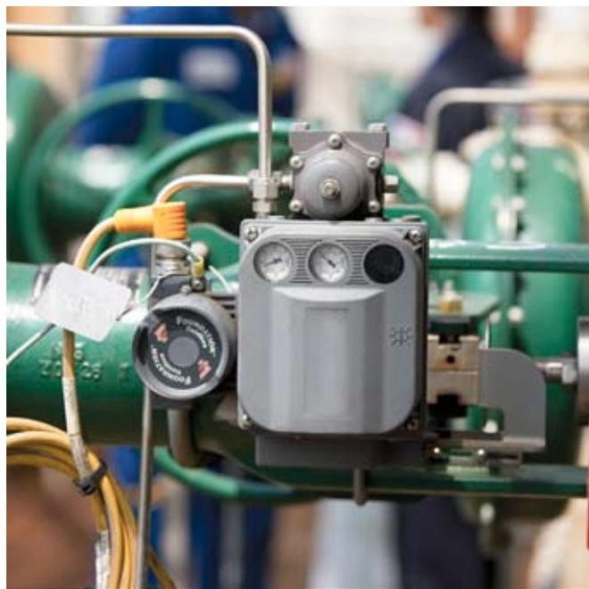
**FIG. 3** Intelligent digital valve controllers provide diagnostics to speed repairs.
