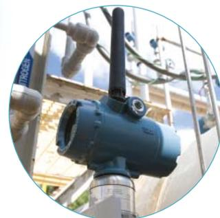
▲ **Figure 2.** Wireless transmitters are recognizable by their radio-frequency antennas and absence of power wiring, which is replaced by onboard long-life batteries.
