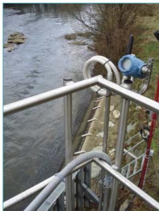
▲ **Figure 5.** Wireless transmitters monitor the returned-water temperatures needed for environmental compliance by a cellulose-fiber producer.
