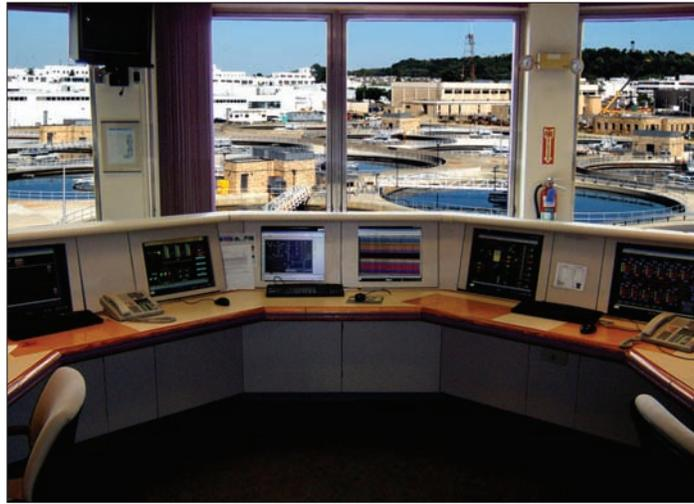
**The integrated control system architecture for water/wastewater industries often incorporates a SCADA system for wide-area monitoring and control of operations from a single location. These operations may include remote pumping stations, wastewater collection systems, water distribution, sewer diversion, wet weather overflow protection, and weather monitoring. Photo by Emerson Process Management**
