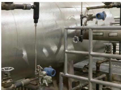
Figure 3. These two Rosemount 3051S multivariable transmitters are each sensing temperature and pressure, and transmitting this and other information back to the host control system via FOUNDATION Fieldbus.
