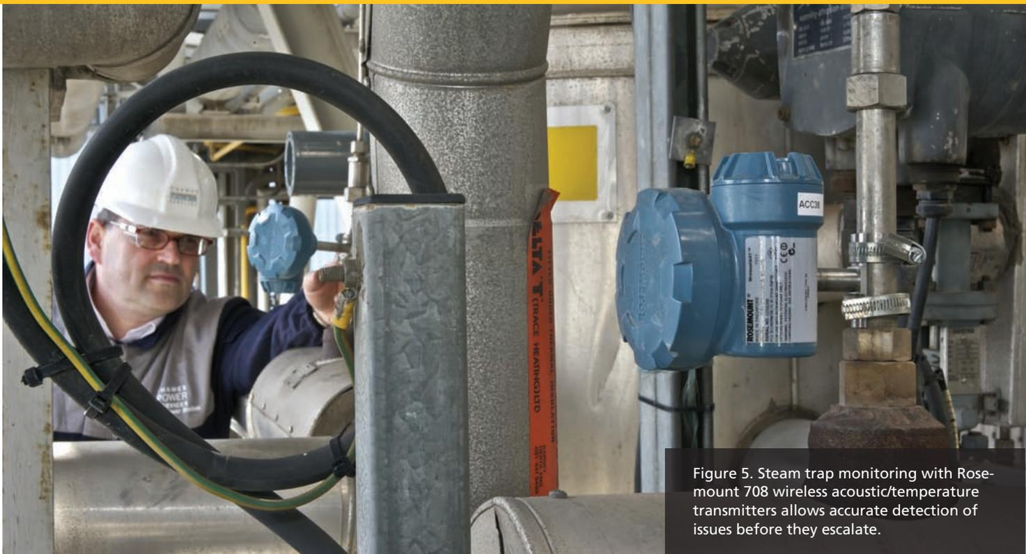
Figure 5. Steam trap monitoring with Rosemount 708 wireless acoustic/temperature transmitters allows accurate detection of issues before they escalate.
