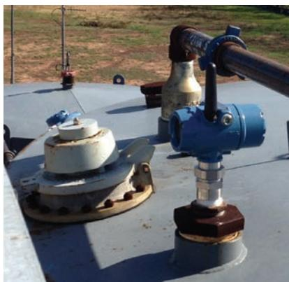
**Figure 3:** Battery-powered field devices, such as this WirelessHART level sensor, can be used in hazardous environments, including tanks containing flammable materials.
