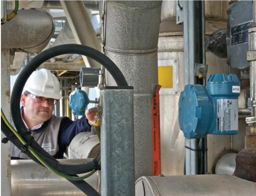
**Figure 2:** Instruments and wiring systems in hazardous locations must be inspected regularly. During a visual inspection, a certified technician looks for obvious faults.
