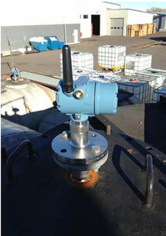
*Figure 1. This wireless guided wave radar device is being used to measure tank level, an application particularly well suited for wireless as connecting a wired device would be difficult due to the hard to access location. (Courtesy of Emerson Process Management)*
