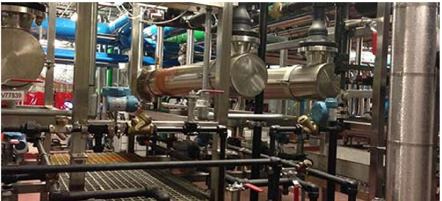
*Figure 2. Wireless instruments can be used to monitor variables on equipment such as heat exchangers, pumps and piping systems. (Courtesy of Emerson Process Management)*
