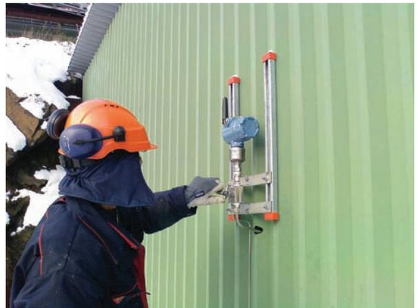
*Rosemount® wireless pressure transmitters provide measurements from the underground storage rooms.*
