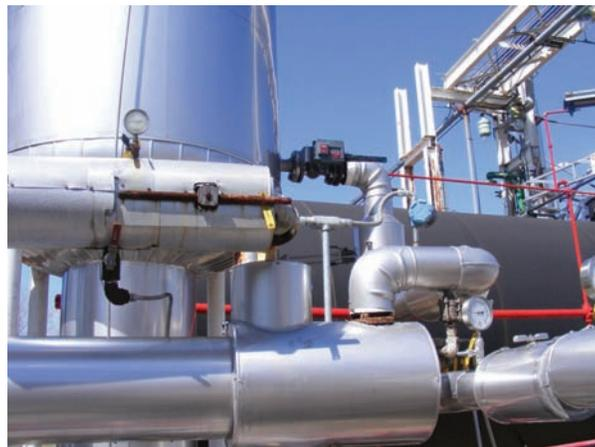
*The Fisher 4320 wireless position monitor installed in the Ethylene Oxide unit is about twelve feet off the ground.*
