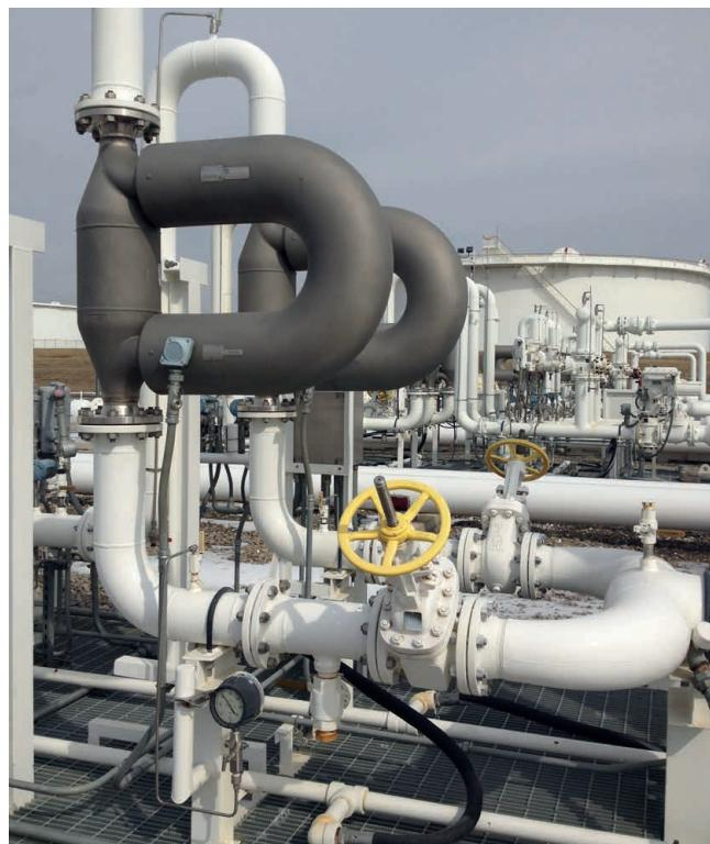
**Figure 4.** The gray U-tube design of each of these two micro motion coriolis meters are clearly visible at this pipeline receiving station for a major storage terminal in Cushing, Oklahoma.
