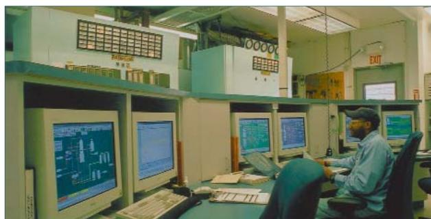
**Figure 7. The operator stations in the control room consist of dual monitor PCs running Windows NT. Parts of the superceded pneumatic control panels are seen**
