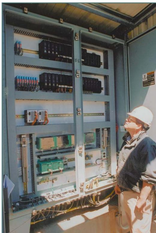
**Figure 4. Authour Verret inspects a field enclosure containing the DeltaV controllers for the naphtha stabiliser (top rack) and Crude Unit 1(second rack).**
