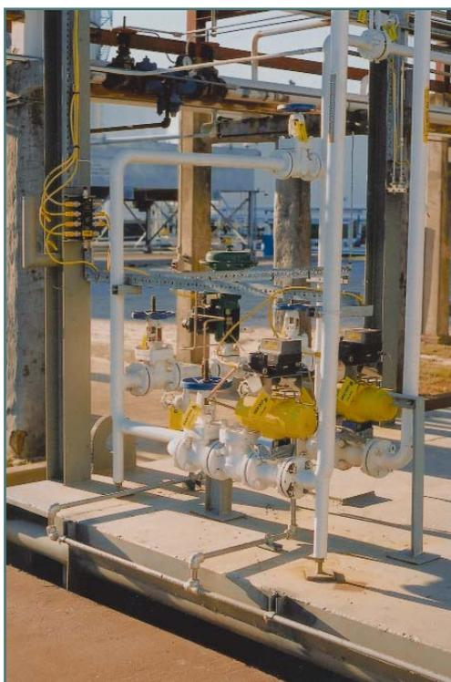
**Figure 6. Fisher controls intelligent DVCs (digital valve controllers) on two switching valves (foreground) and one throttling control valve (further back). They communicate and receive power through a FOUNDATION fieldbus segment, via flexible yellow cables with weather tight, quick disconnect fittings and the branch block on the column.**
