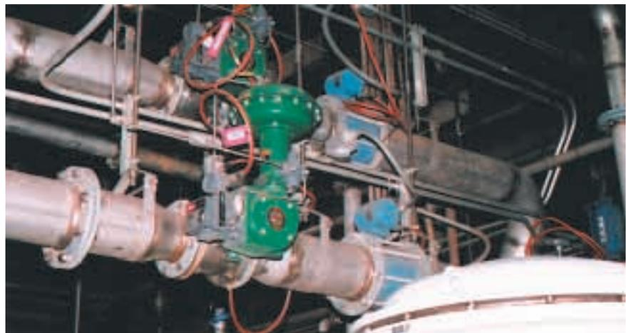
Valves with digital valve controllers and intelligent magnetic flowmeters connected via Foundation fieldbus
