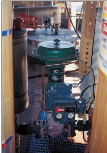
DIGITAL CONTROL VALVES AND DIAGNOSTIC SOFTWARE ALLOW QUICK AND PRECISE RESPONSES TO SIGNS OF VARIABILITY TO ELIMINATE PROBLEMS BEFORE PRODUCTIVITY IS IMPACTED.
