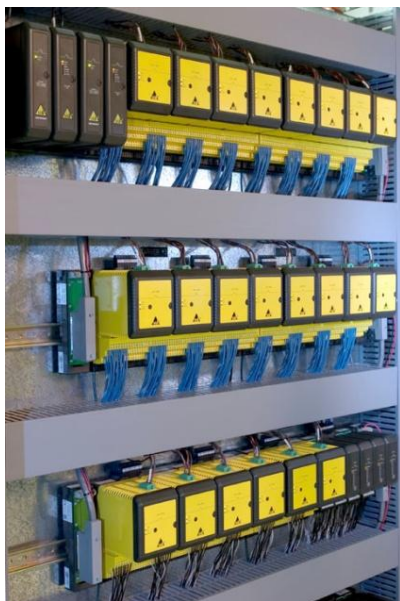
DeltaV SIS logic solvers mounted horizontally
