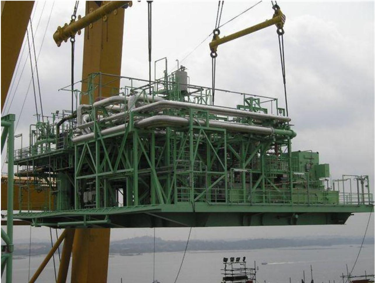
*A fully constructed Module complete with system cabinets and signal wiring is hoisted onto a main structure*
