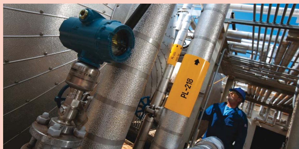
Smart Wireless transmitter monitors BP tank farm.
