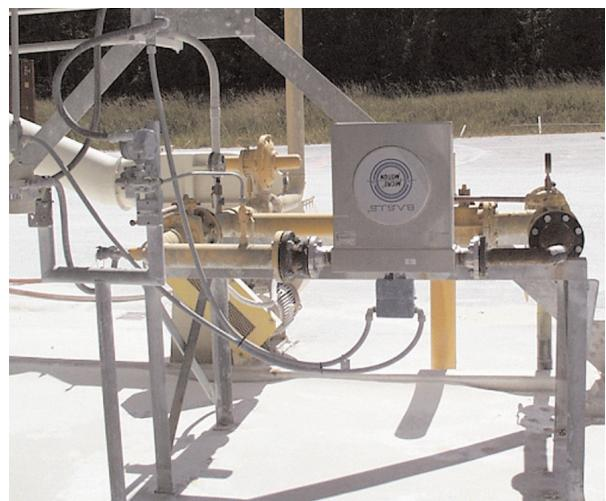
*Micro Motion meters prove less expensive and easier to install than traditional gas measurement technologies.*
