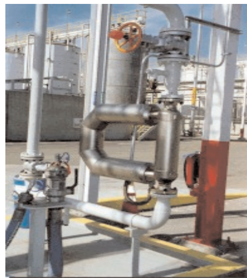
Micro Motion batches reactor products into tank trucks.
