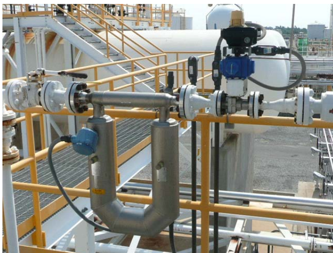
Micro Motion ELITE (CMF200) with MVD and Smart Meter Verification technology.
