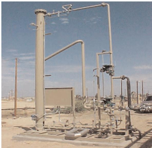
*Two Micro Motion Coriolis flowmeters replace costly three-phase test separators, enabling an oil producer to conduct accurate daily well tests.*
