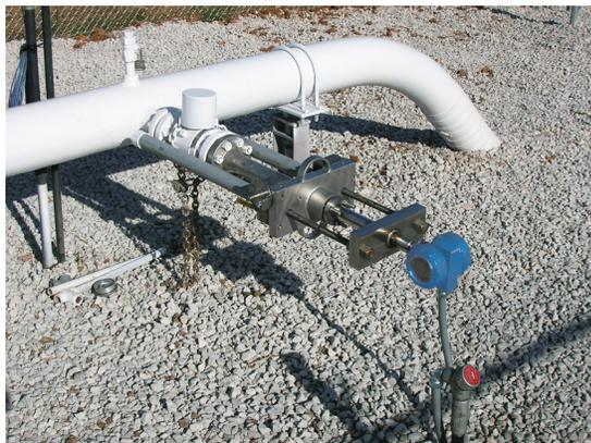
**Installed retractable fork density meter**
