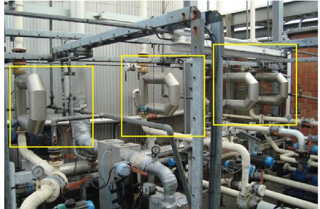
ELITE CMF300 meter pictured in vertical flow upwards, operating in harsh entrained gas and vibrational conditions.
