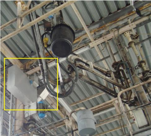
To the left: a CMF300 insulated, in flag position, flowing upwards.
