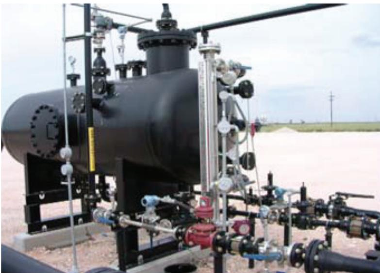
*Installation of a three-phase test separator*
