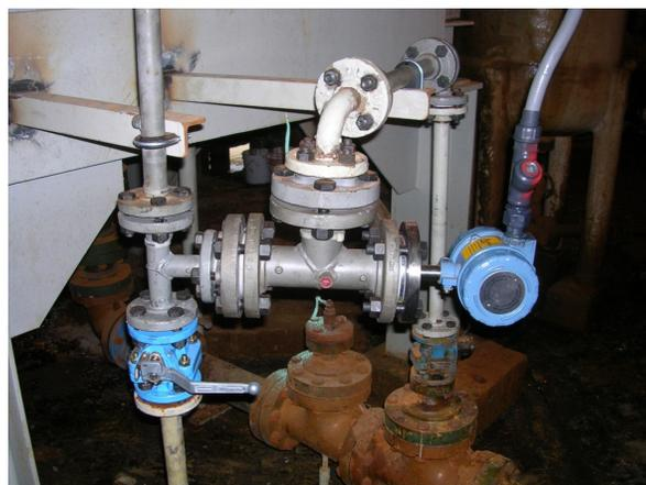
*Installation of a Micro Motion insertion liquid density and concentration meter in Zirconium at the silicone manufacturer*
