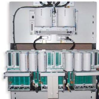
This image depicts one crate of 12 Q-Line cards migrated to Ovation I/O. The original card edge connectors are plugged into the personality modules. The picture also shows the Ovation controller with the power and communications cables.
