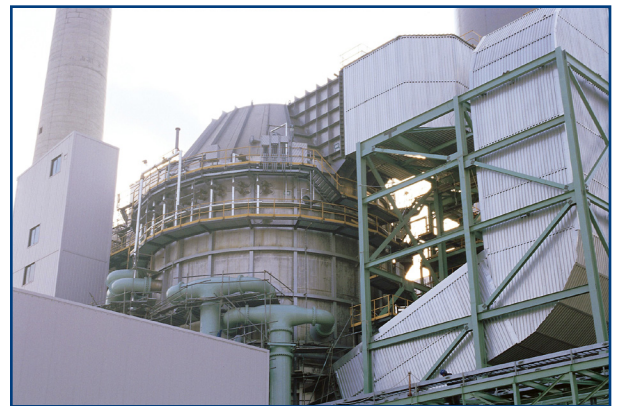
Use of technologies like a flue gas desulphurization system helps to secure Yonghung's place as one of the most clean and efficient power plants in the world.
