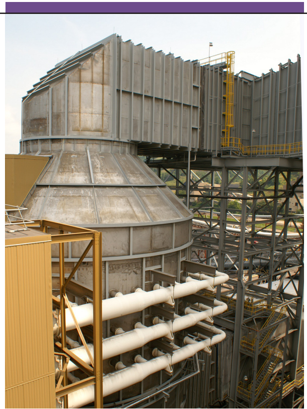
Absorber vessels, as shown above, were installed for both Mitchell units as part of the new FGD systems. The logic for this equipment was incorporated into the plant’s Ovation control system as part of the upgrade project.
