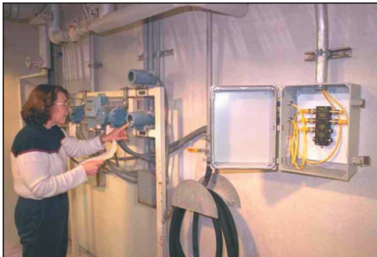
Figure 4. Rosemount FOUNDATION fieldbus transmitters (left) and fieldbus segment connector block (right).
