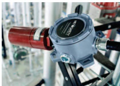
**Triple infrared (IR) flame detectors offer the highest level of immunity and maintain a very fast response with wide area coverage**
