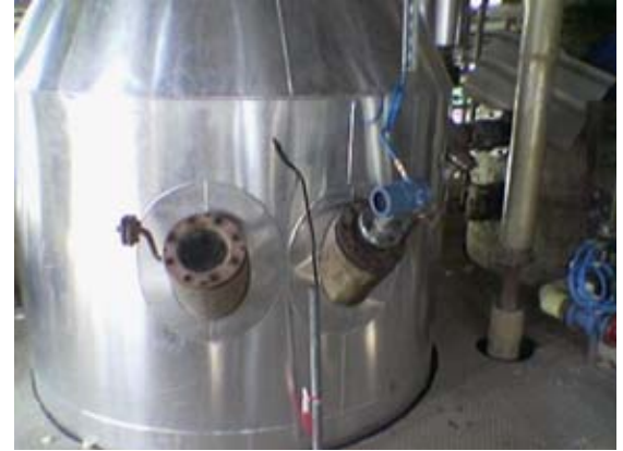
Inclined installation at 35° of Rosemount 3300 gives the customer a reliable level reading from a non-standard tank shape.
