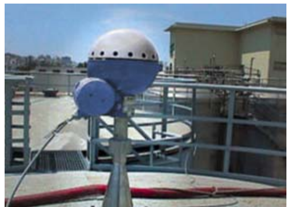
The Rosemount 5600 transmitter is mounted on an existing nozzle on the tank roof.
