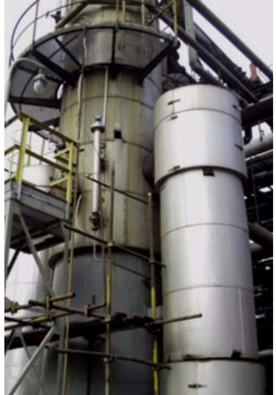
Rosemount 3300 reliably measures the level in a methanol distillation column.
