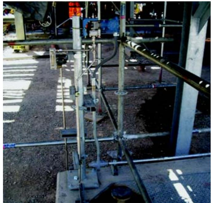
*In addition to the necessary control loop connections and process mounting, a bubbler system also includes an air supply with filter regulator, tubing and fittings to the transmitter, a rotometer for regulation of the air supply and a mounting support for the transmitter.*
