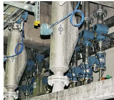
Rosemount 8700 Magnetic flowmeter systems and Micro Motion F-series Coriolis meters precisely measure ingredients in Stora Enso's Coating Kitchen.
