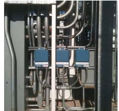
Three Smart Wireless Gateways communicate to 75 wireless devices up to 1500 feet away.
