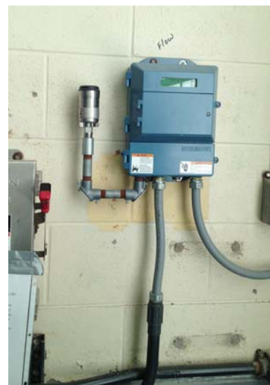
Wireless THUM Adapters bring stranded flow measurements on-line, and eliminate the need for manual totalization.
