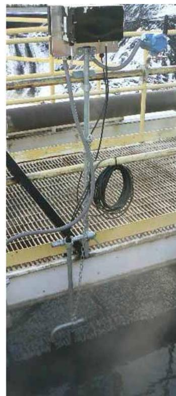
*Mobrey MSL600 Sludge Blanket Level Monitor and Rosemount 648 Wireless Temperature Transmitter*
