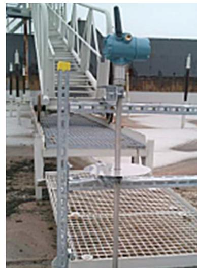
*Use of wireless vibrating level switch for floating roof monitoring.*
