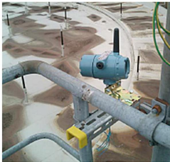
*The use of a repeater ensures the wireless signal from the Rosemount 2160 is transmitted to the Gateway when the roof is at a low level.*
