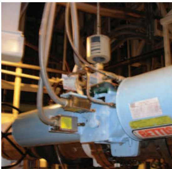
Pneumatic rotary actuators installed in a nuclear power plant.
