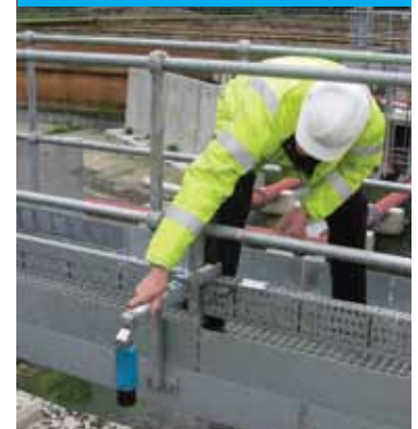
3107 Pumping station level
