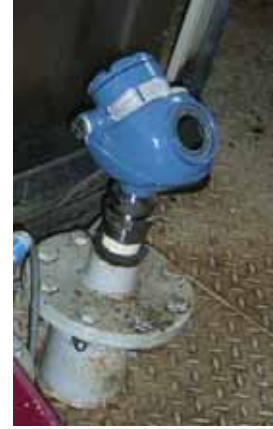
Figure 2. Installation of Rosemount 5303 Guided Wave Radar.
