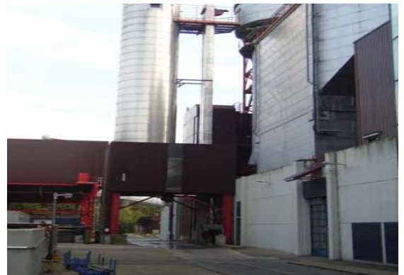
Figure 1. 60-ft (18.5 m) tall combustion salt silo at garbage incineration plant.
