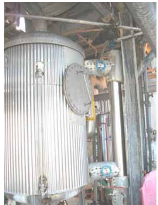
Figure 1: Installed Rosemount 3301
