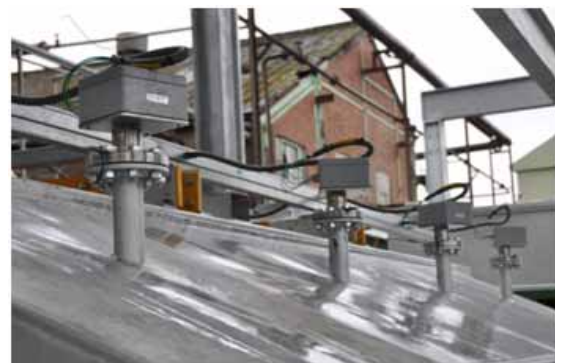
Figure 1. Installed Rosemount Multipoint Application and Industry Solution (AIS) sensor
